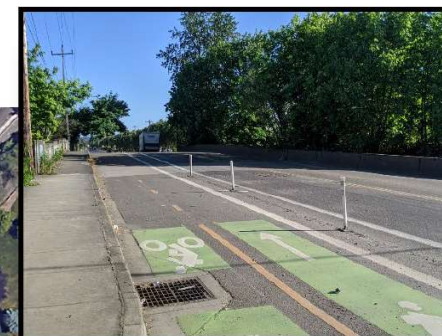
Figure 1: Jersey barriers line the west side of the existing bridge
