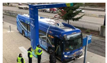
Beaverton Transit Center Overhead Pantograph Fast Chargers
