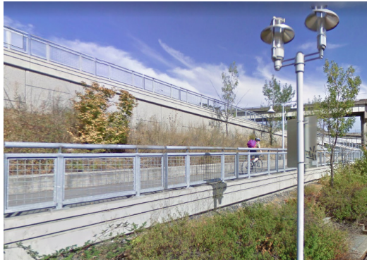
Example of multi-slope concrete ramp and MSE retaining wall approach structure
