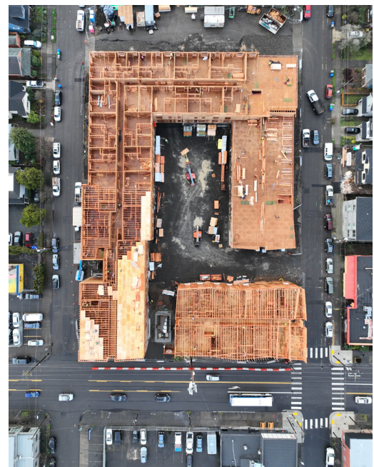
Glisan Landing Under Construction | Portland
