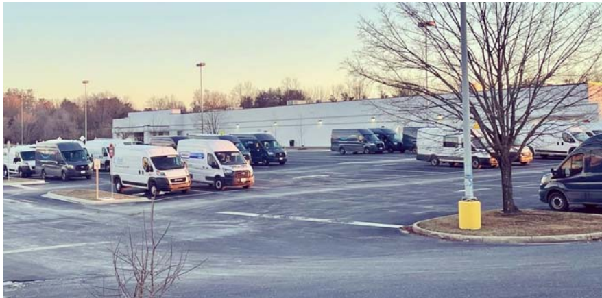
Figure E.8 Conversion of a former Kmart “Dark Store” to an Amazon Delivery Center in Waynesboro, Virginia
