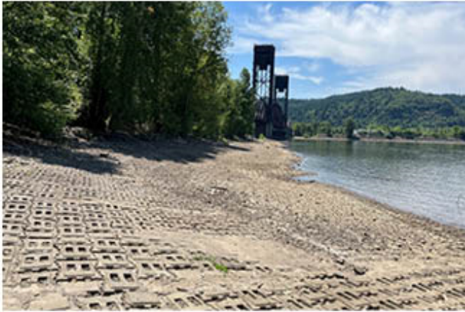
Photograph 1: Shoreline - concrete block armored cap Facing South Location: East Parcel Year: 2023
