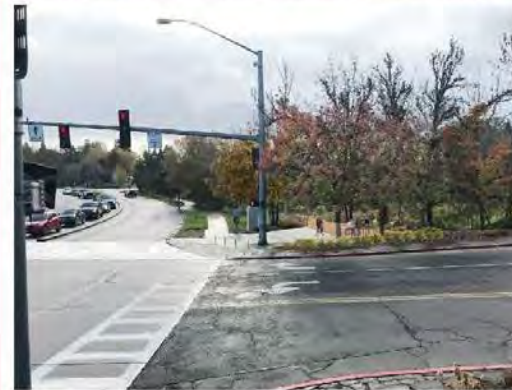
C6B: Plaza Area at Dartmouth Street/Costco Driveway
