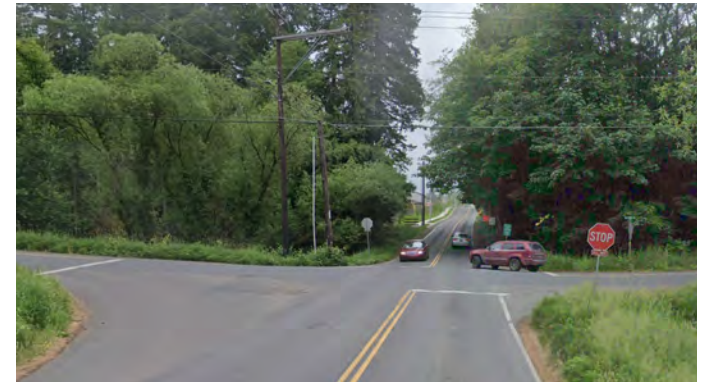
SW Edy & SW Elwert intersection (Significant improvements are needed)
