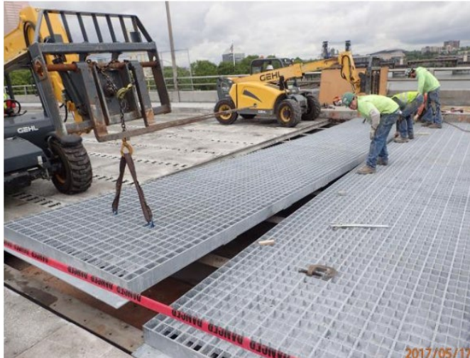
Installing new steel grate deck on the Morrison Bridge. Photo courtesy of Multnomah County
