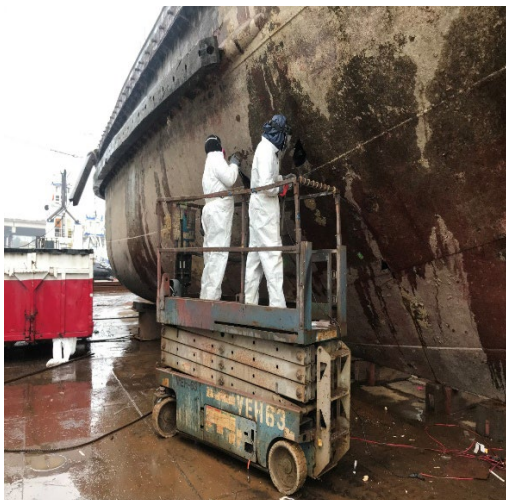
Sakarissa – Sawzall Access Cut to Hull in Progress
