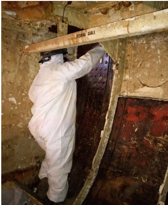
Certified Abatement worker scrapping PCB-Lead Paint
