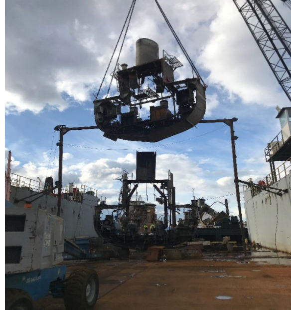
DB Freedom – Lifting 35-ton piece from DD-2 to Barge
