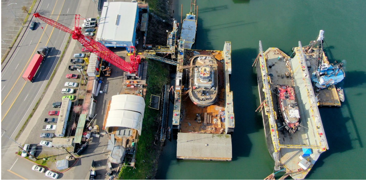
Looking from Overhead with Dry-dock No. 2 to shore and Dry-dock No. 4 outboard.
