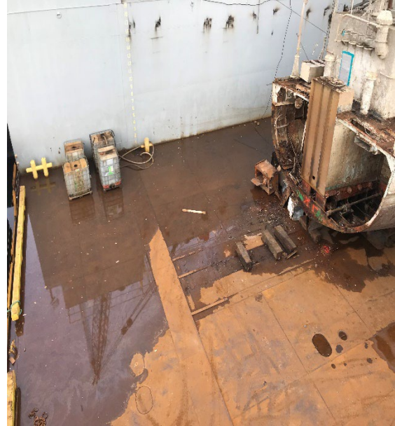
Overhead view at Lower Sump of Totes and Pump/Hoses
