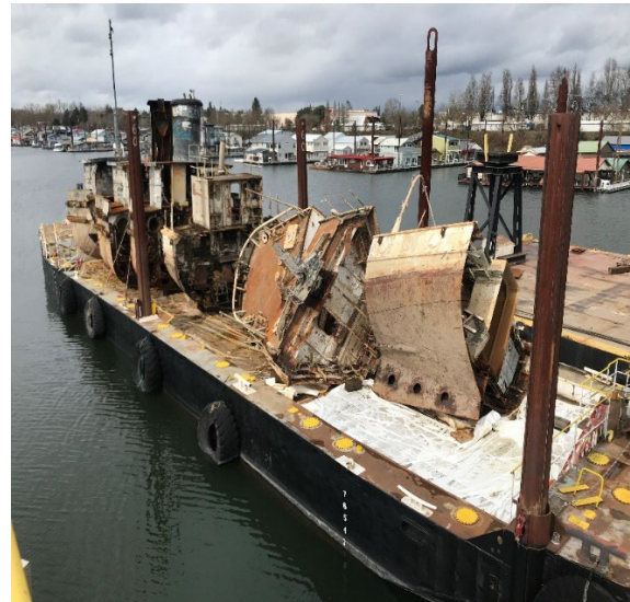
R-22 – Barge Secured and Ready to Transport to Recycler
