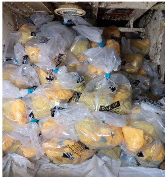
Asbestos – Haz Waste Double Bagged on Vessel
