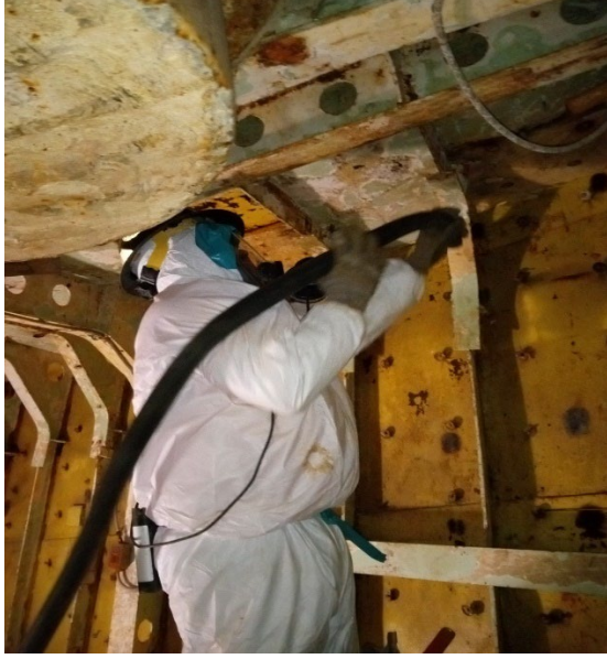
Certified Abatement worker vacuuming PCB-Lead Paint
