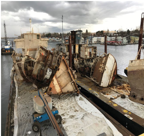
R-22 and JBT-09 – Barges being filled with vessel scrap pieces.
