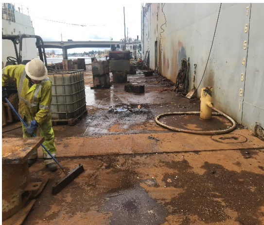
DD-2 Typical Deconstruction Waste Cleanup
