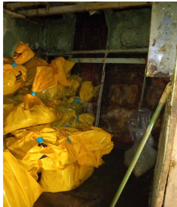
PCB-Lead Paint & Debris Collected in Special Bags
