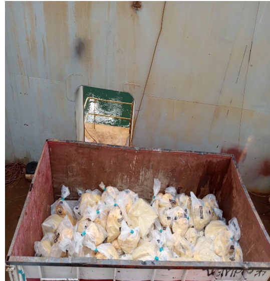
Asbestos – 20-Yard Container on Drydock
