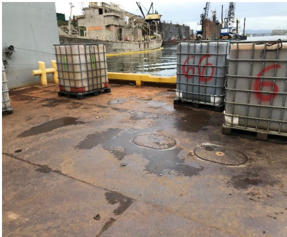
Full Wastewater Totes Ready to crane off Drydock
