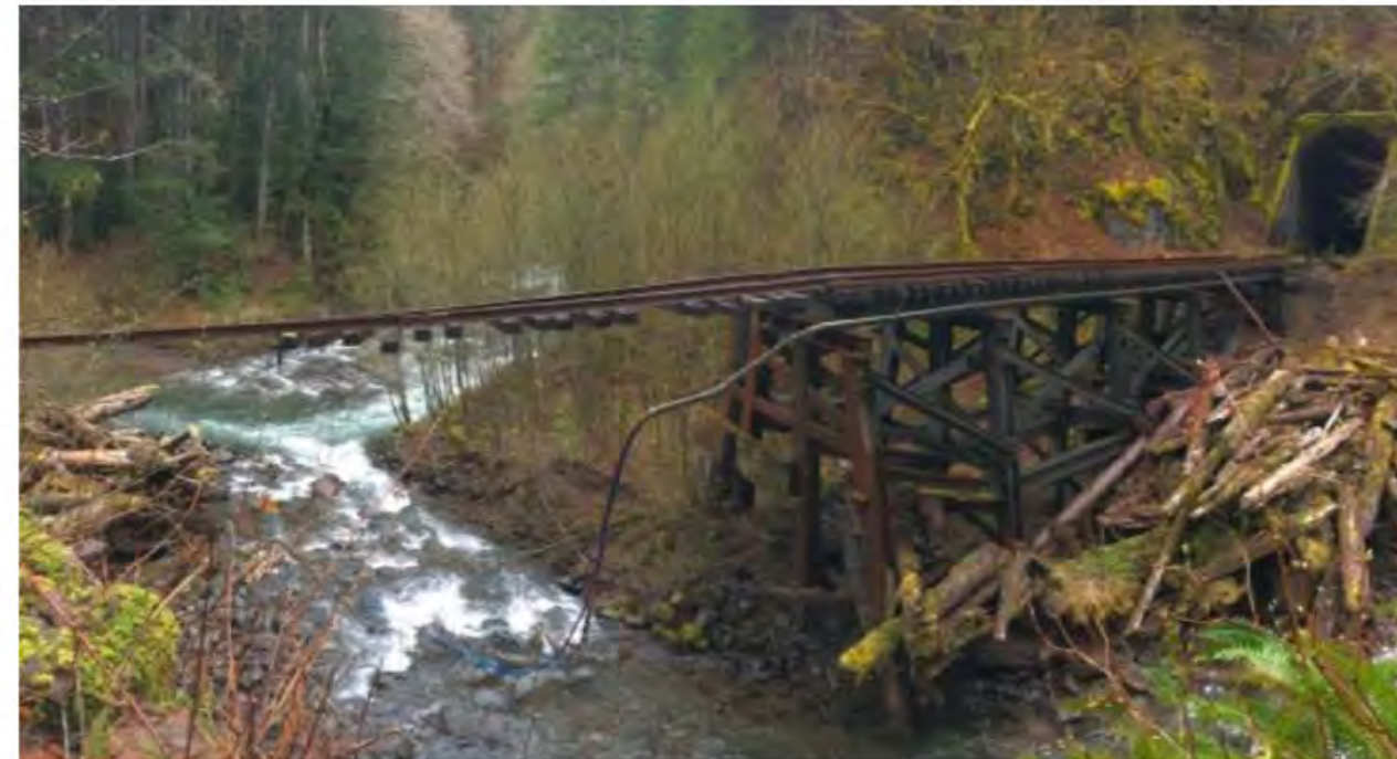
Photograph 1-7. Kinney Creek Tunnel-Collapsed Trestle (2018)
