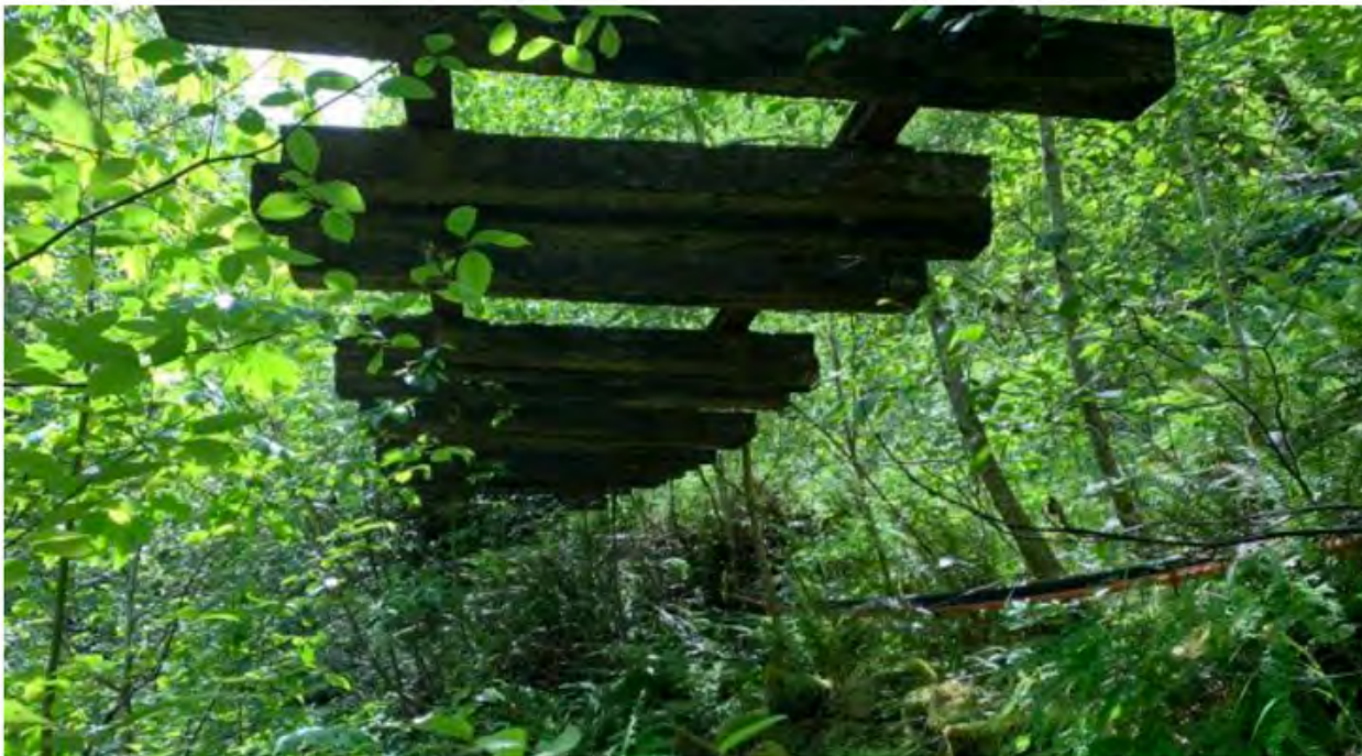
Photograph 1-6. Rails and Ties in Air (2020)
