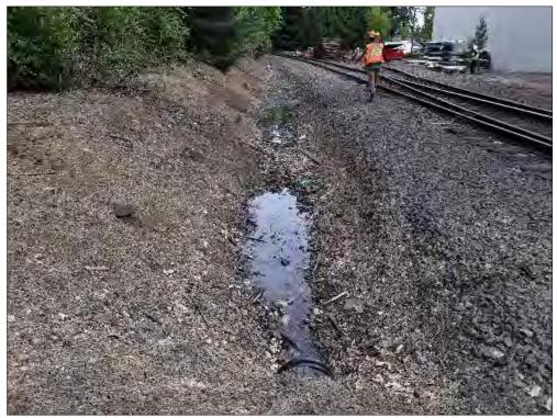
Photo PP-C20: Looking southeast at Railroad Ditch D-Cc from culvert. Ditch is located between railroad berm and adjacent upland slope. Some ponding present during the May 2020 site visit and recent indicators of flow including presence of litter and water staining.
