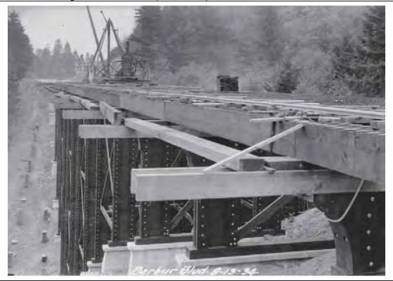
View: SW Newbury Street Viaduct deck and timber trusses under construction, facing south (OSHD 1934g).
