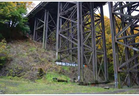
View: South trusses and earthen abutment, facing southwest. The remains of the former railroad trestle footings are at lower left.
