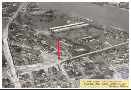
View: A 1948 photograph of the reconstructed west approach to Ross Island Bridge, near completion. Note the different shape and alignment at the end of the west approach (at arrow) to accommodate curving on- and off-ramps of the bridgehead. The view is towards the north-northeast. City of Portland (OR) Archives, A1999-004-1107.
