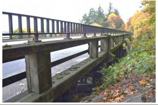
View: SW Vermont Street Viaduct west rail detail, facing southeast. Note the missing balusters.
