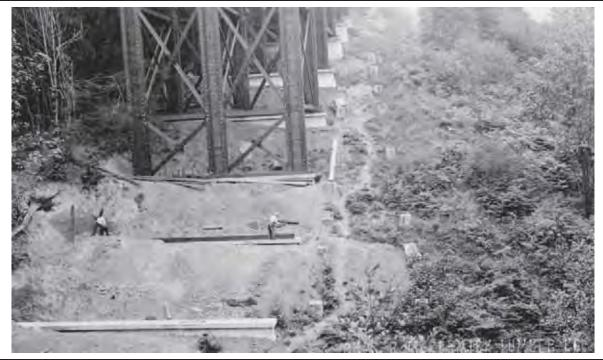
View: Viaduct footings and substructure under construction (OSHD 1934f). At right, note the remnant footings of the former railroad trestle that predated the viaduct.
