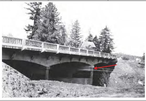
View: Circa 1935 image of the Oregon Electric Railway Overcrossing. The red arrow points to where electrical transmission lines were attached to the north bridge bent; an insulator remains at this location in the present day. Photograph courtesy of the Oregon Department of Transportation (02010 004).
