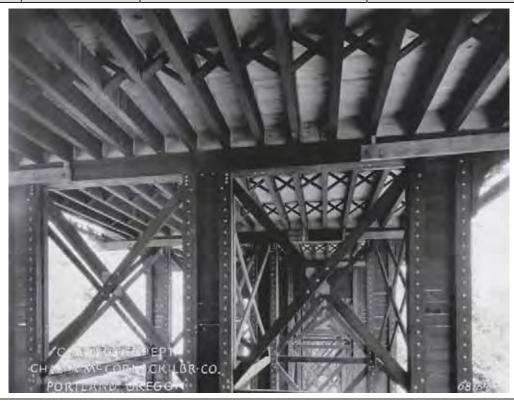
View: Timber truss and stringer details under deck (OSHD 1934f).
