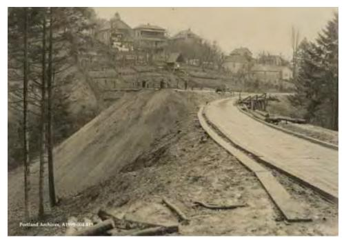
Photo 5-5. Construction of SW Barbur Boulevard at an unnamed gulch near SW Hamilton Street in 1932. The likely remnants of a wood railroad trestle are visible at right; the curving alignment at right is likely that of the former Southern Pacific electric interurban line that was removed for road construction. City of Portland (OR) Archives, A1999-004.419.
