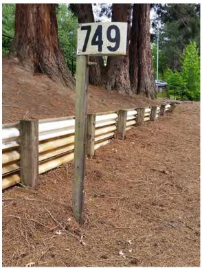
Photo 7. Mile marker 749 along the SPRR Tigard Branch is part of the historic resource. The wood post was originally a telephone pole crossarm. Note the intact threaded wood peg to secure an insulator directly below the metal sign. The view is towards the southeast.
