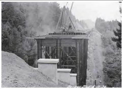
View: Concrete footings and timber substructure under construction, facing north-northwest (OSHD 1934c). Remnant footings from the railroad trestle that predated the viaduct are at right.
