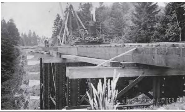
View: Pressure-treating timber stringers during viaduct construction (OSHD 1934e).
