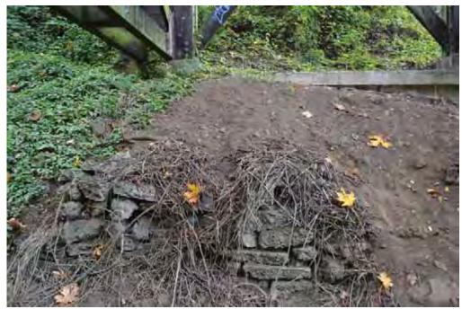
View: Concrete rubble support in earthen abutment near concrete footing, facing north.
