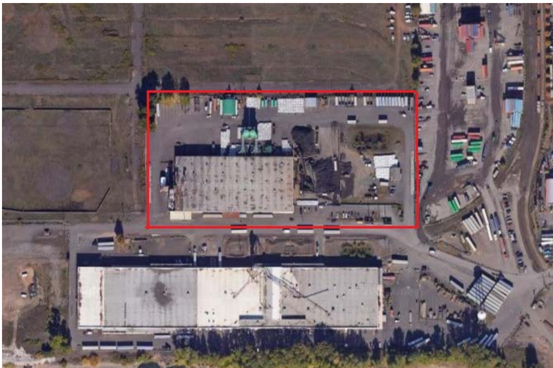
Aerial view of the RB Recycling facility
