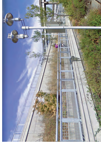
Example of Multi-slope Concrete Ramp and MSE Retaining Wall Approach Structure
