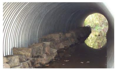
Not all wildlife crossing budgets have big price tags. This rock shelf was constructed in a culvert in Loraine, Oregon to provide passage for terrestrial wildlife when water is in the culvert. Photo credit: John Levenhagen.
