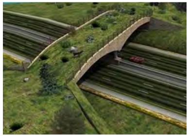
Figure 5-41 This is a graphic rendering of the wildlife overpass proposed for I-70 west of Vail Pass in Colorado. Graphic credit: Digital Animation Services.
