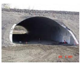
Figure 5-13 The underpass on S.R. 240 in Washington was constructed for about \$700,000 and was built for deer, coyote, and other small mammals. Photo credit: Washington Department of Transportation.
