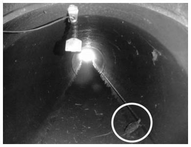
Terrestrial wildlife will use culverts that pass water if an elevated concrete walkway or shelf (preferably at least 18 inches wide and 12 inches high) is constructed along the inside of the culvert (Figures 5-19, 5-20, 5-22, 5-23, 5-24, 5-25). Culverts that pass water and have no shelving may be barriers for some species (Figure 5-21).
