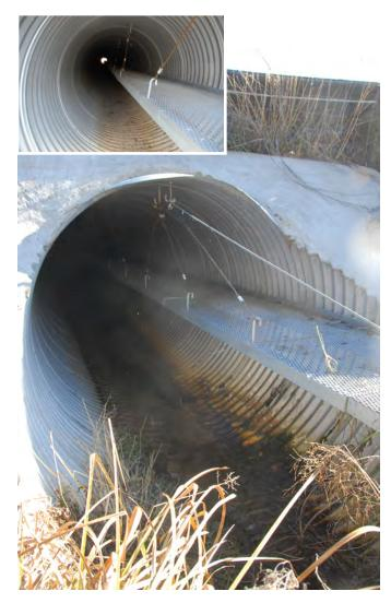
The Critter Crossing<sup>™</sup> structure was placed inside this drainage culvert under U.S. 93 between Stevensville and Florence, Montana. Suspended shelves allow small mammals safe passage throughout the year. Some of the culverts carry water 4-6 months per year, while others carry water year round. Photo credit: Kerry R. Foresman.
