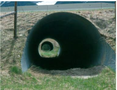
Figure 5-42 This upland culvert is one of many wildlife crossing structures on the Trans-Canada Highway constructed primarily for elk, deer and moose. Photo credit: Scott Jackson.
