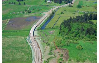
Figure 5-1 The Boeckman Road Extension Project in Wilsonville has elements of a successful wildlife crossing. There is an elevated bridge over a wetland, native vegetation plantings, fencing and land ownerships to maintain the wildlife corridors in perpetuity. Photo credit: Lisa Nead, City of Wilsonville.
