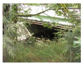
this roadway). A recently renovated bridge over Johnson Creek now has steep, almost vertical concrete slopes on both sides underneath the bridge, preventing terrestrial crossings of any kind. This structure presents an opportunity for retrofitting to enhance wildlife passage. Photo credit: Lisa DeBruyckere.
