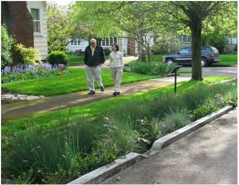
Stormwater Bioswale (Natural detention and filtration of on-street rainwater)
