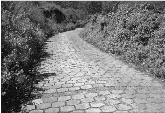
Sand set permeable pavers.
