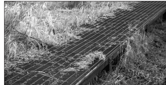
Metal grates can provide a dry trail through a wet section.
