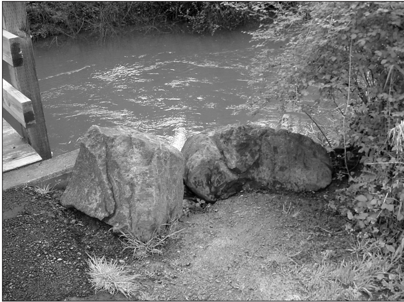
A social trail leading to the stream is obliterated by placing big boulders at the end of the steep trail.
