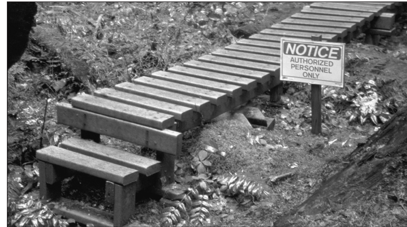
A duckboard elevates the tread surface above a wet area.
