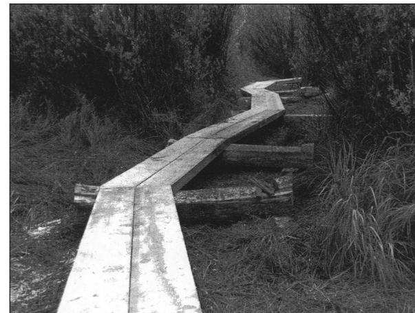
Log supports laid flat on the ground provide a foundation for a low-use bog bridge while limiting disturbance to a fragile wet area. (Wetland Trail Design and Construction, 2001)
