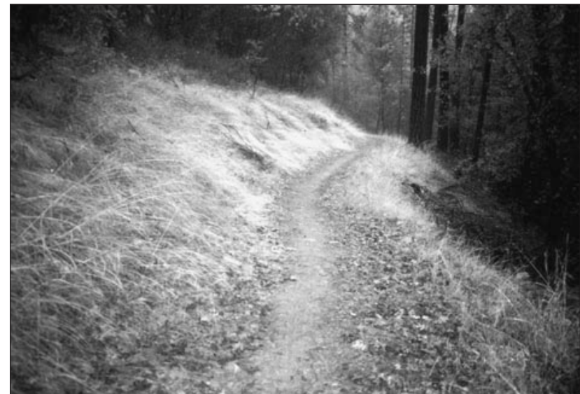
In this road to trail conversion a former forest road was ripped, reshaped and seeded. (Heavy Equipment Operator's Guide to Road Rehabilitation, Casaday and California Department of Parks)
