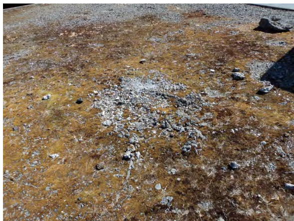
Photo #3 Close-up photograph of the concrete and gravel fill material observed on the Property.
