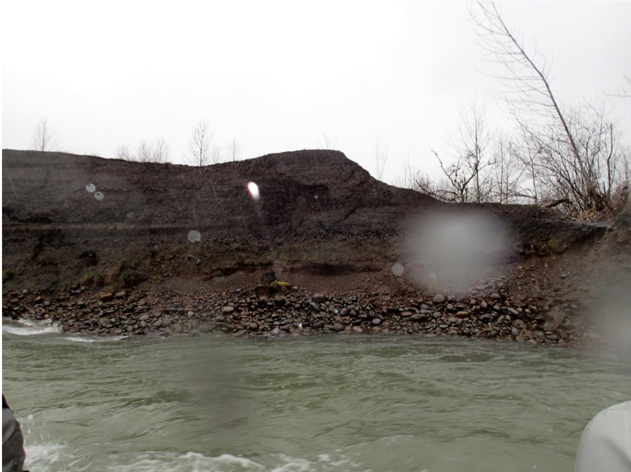
Figure 13 Right bank borrow area. Compacted gravel and quarry remnants visible above alluvium.
