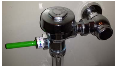
Dual-flush valves at Antoinette Hatfield Hall will help save 420,000 gallons of water a year.
