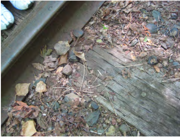
PHOTO 5-1: RAILROAD TIE WITH DATED NAIL HEAD
