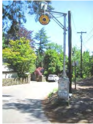
PHOTO 5-5: WIG-WAG CROSSING SIGNAL AT SW RIVERWOOD ROAD
