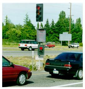
*Ramp metering reduces the delay associated with traffic merging onto freeways.*
