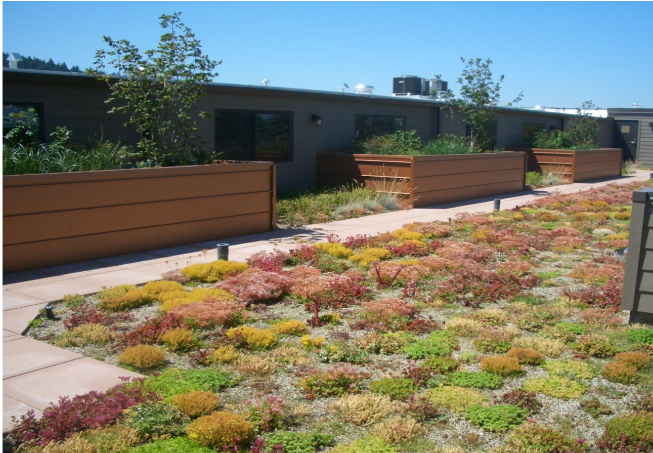
Flow-Through Planters and Green Roof
