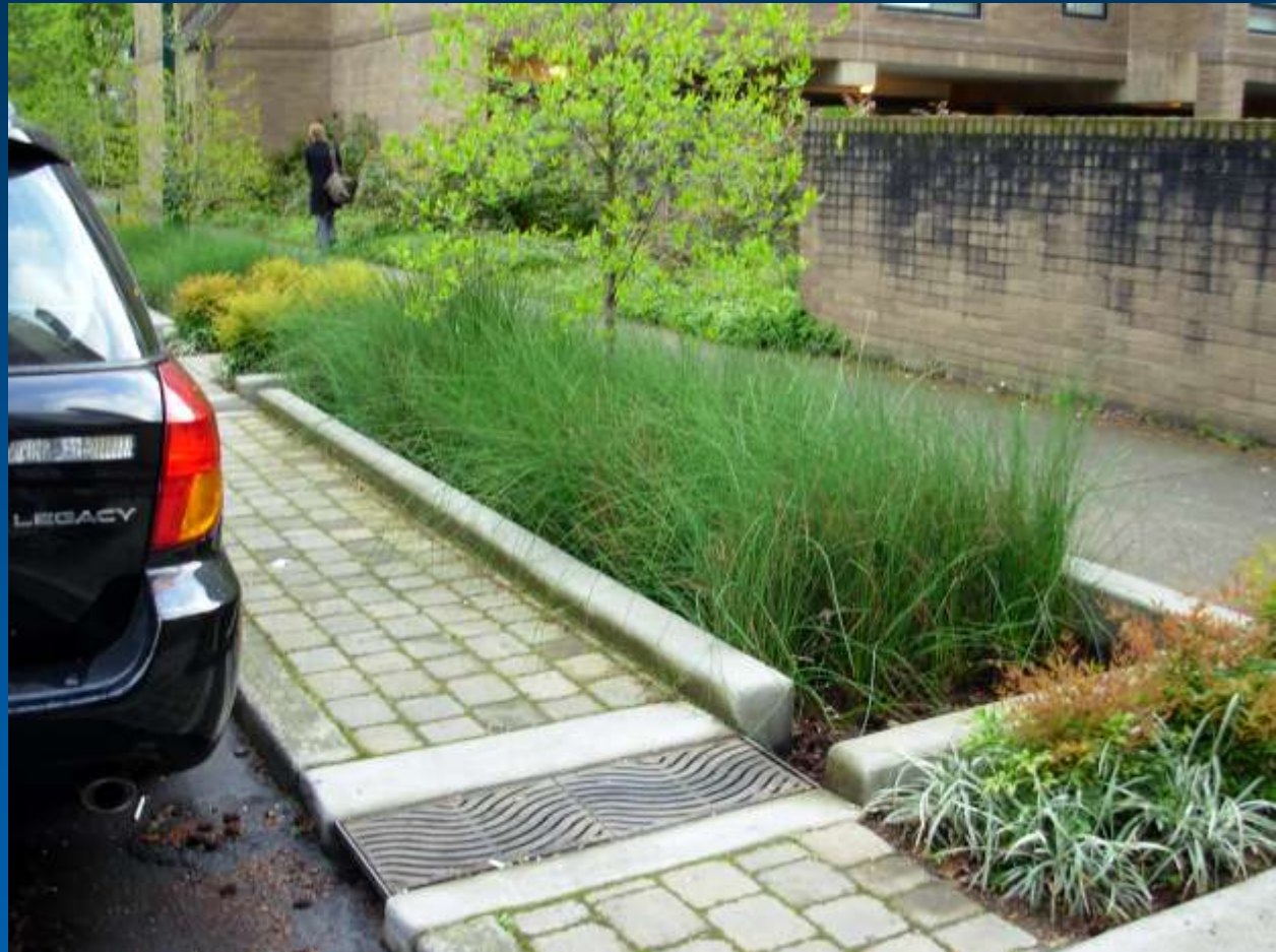
PSU Stormwater Planters
