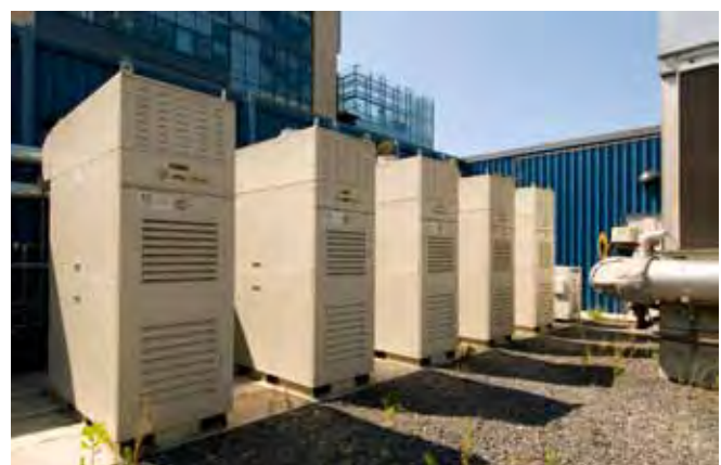
Microturbines at OHSU-South Waterfront
