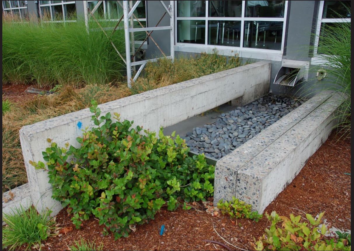
A roof drain integrates into the landscape as a flow-through planter.
