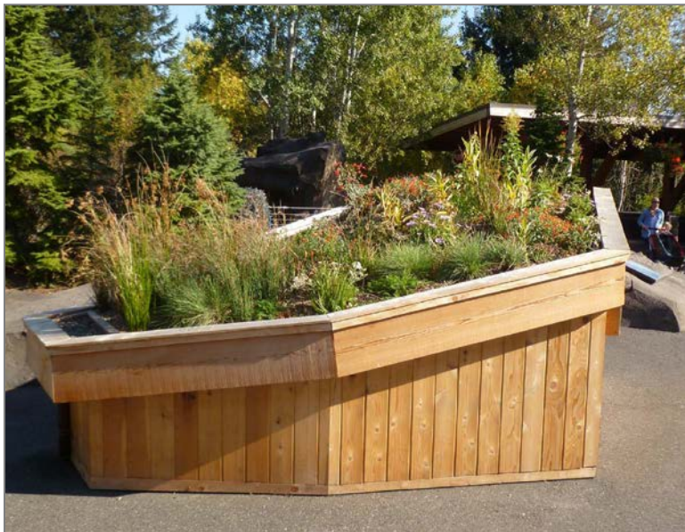
A model ecoroof at the Oregon Zoo tests a steep slope technique and educates visitors about the benefits of green roofs.
